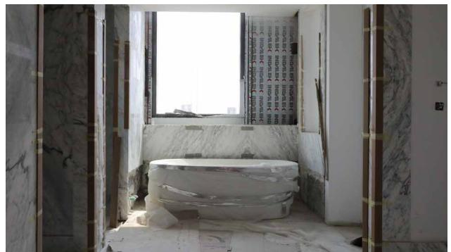
**Master Bathroom**- Marble installation level 3 is done, continuing to level above
