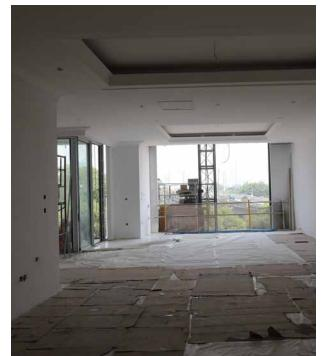
Marble installation for residence is starting. Homogeneous tile installation is in progress at basement 2 to 4 and level 3. Block wall partition installation reaches level 22
