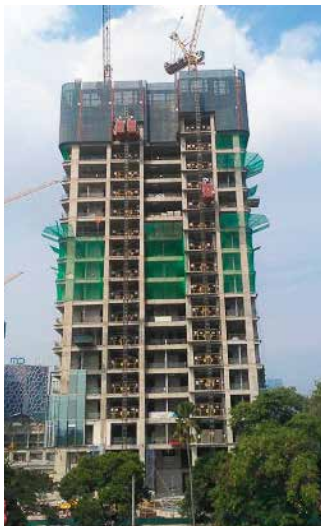
As of June 2019, The Residence structure has reached level 26 to level 27
