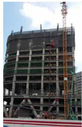
As of July 2019, Office tower for structural works has reached level 15
