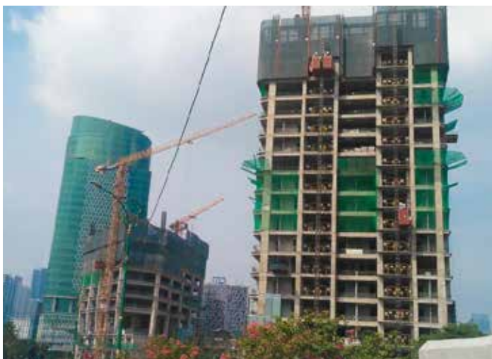
As of June 2019, Office tower structure has reached level 13
